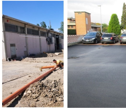
The pavement -before and after
