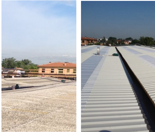
The roof before and after
